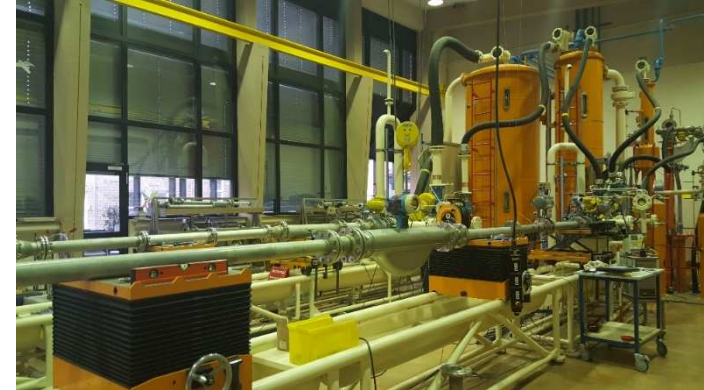
Hydrocarbon flow calibration rig with flowmeter installed in PTB
