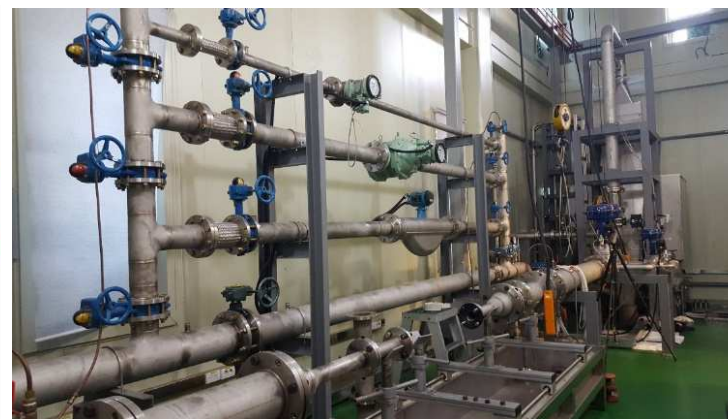
Hydrocarbon flow calibration facility (light oil) in KRISS
